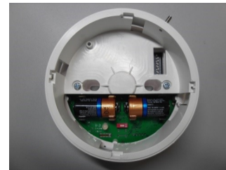
Picture 6 - primary and secondary batteries inserted
