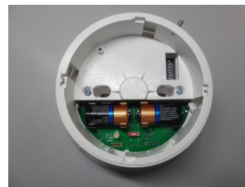
Picture 6 - primary and secondary batteries inserted
